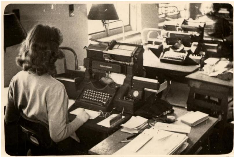
Figure 5: A programmer operating a card punch [2]
